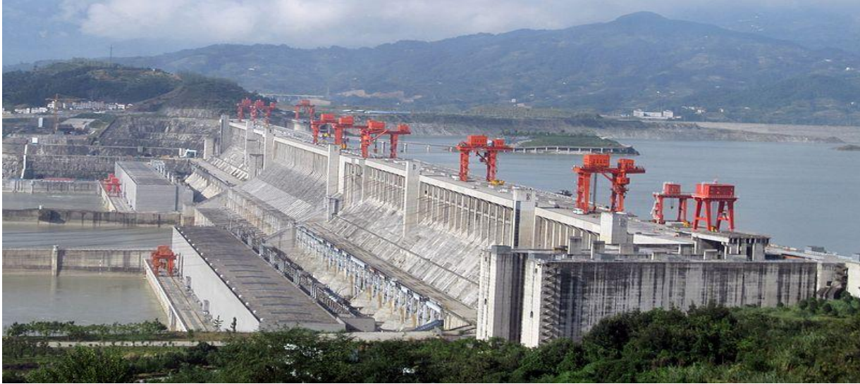
Figure 3.6 The Three Gorges Dam on the Yangtze River in China.
