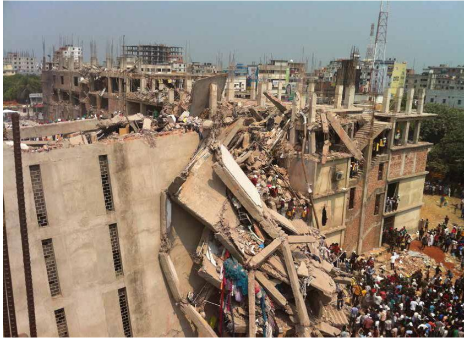
Fig 3.6 Rana Plaza building collapse, April 24, 2013.
