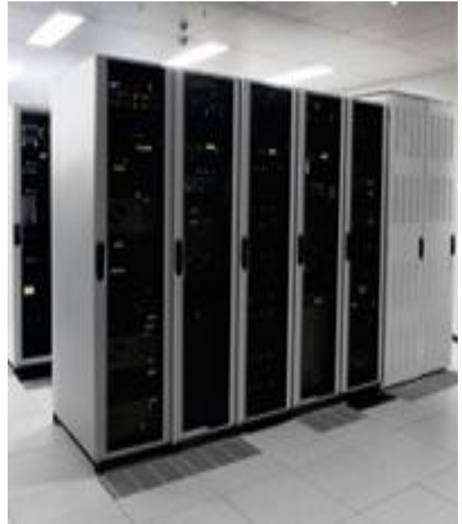
Figure: 6.2 Create & Optimize Data Centers with ETAP
