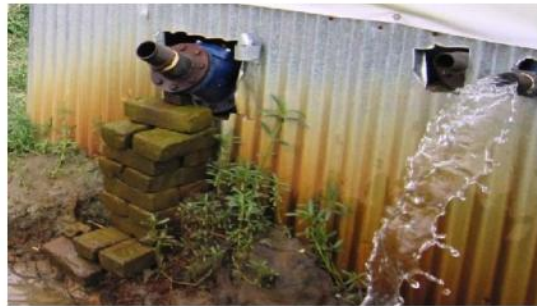
Fig 1.2 Pump Installation in rural area
