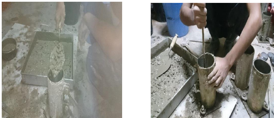
Fig 3.15: pouring and scaling of concrete
