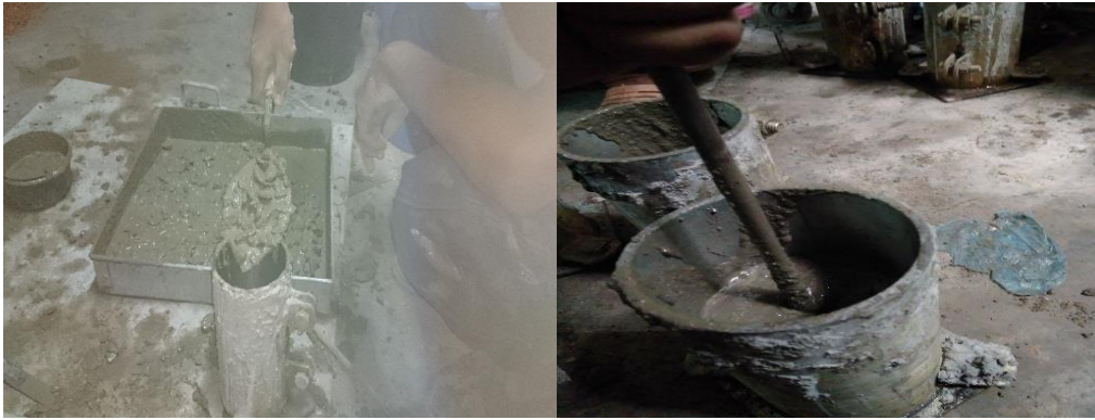
Photo 3.12: pouring and tamping of concrete
