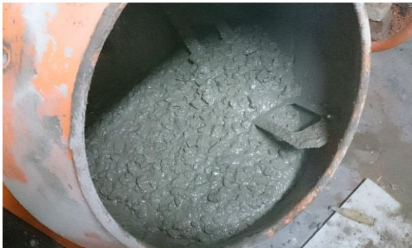
Photo 3.11:Mixing of concrete
