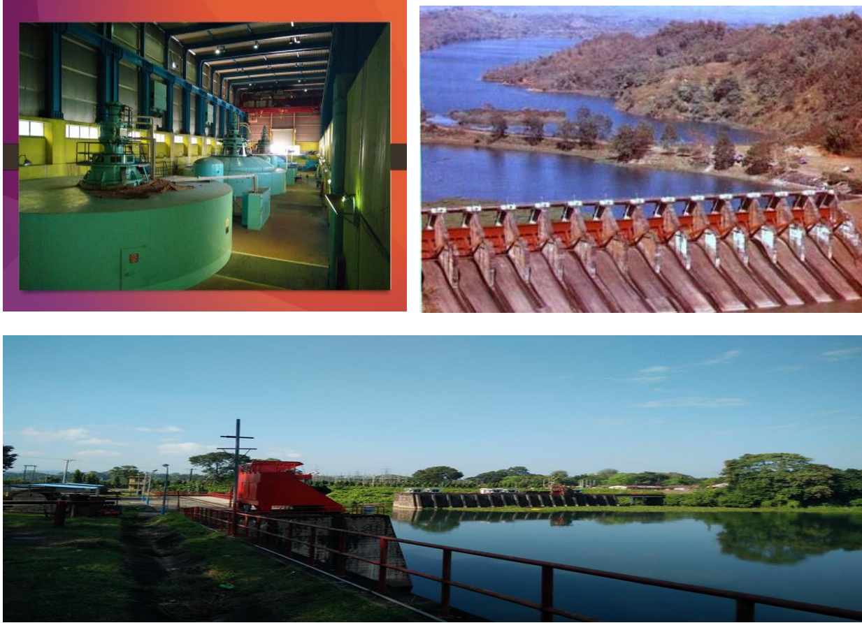
Figure 1: Karnaphuli Hydro-electric Power Plant
