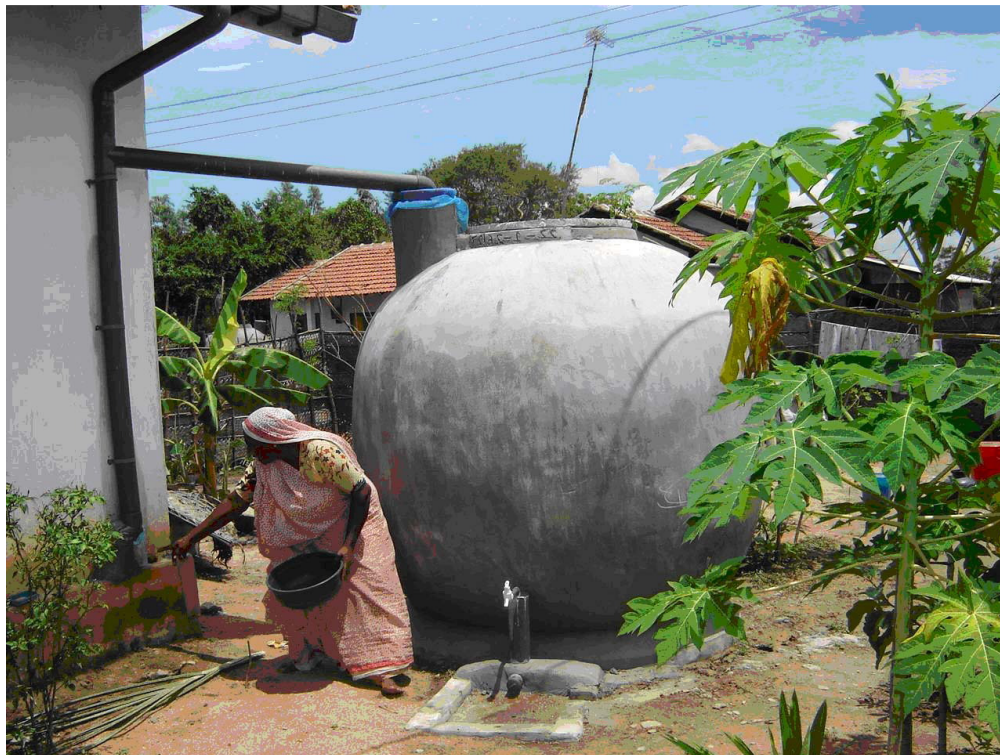
Fig (2.9): water harvesting system
