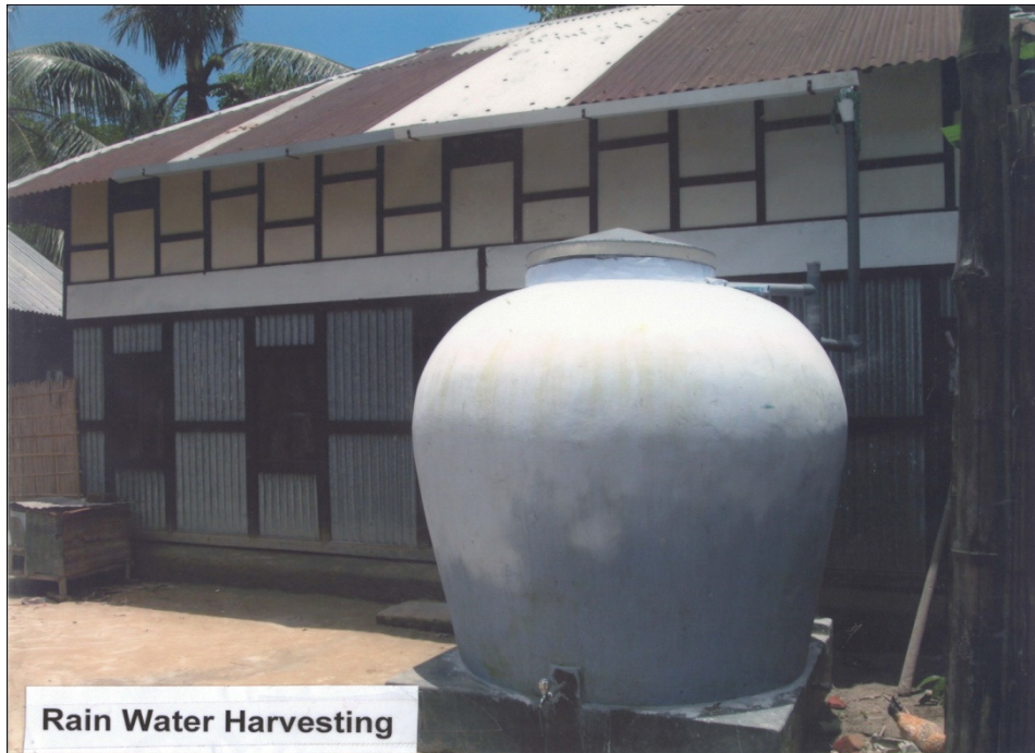
Fig (2.8): water harvesting system
