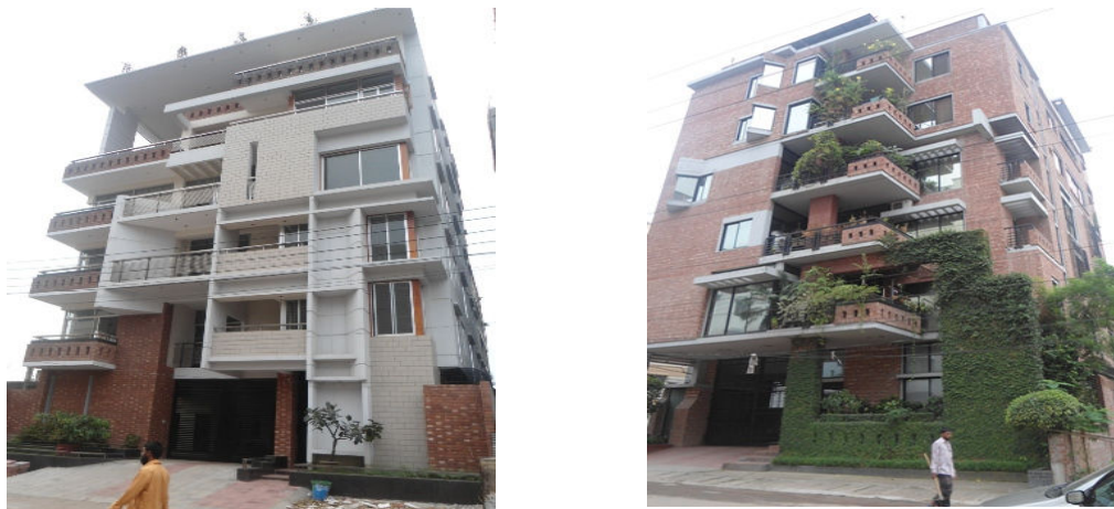
Figure 2.1. RCC frame building.
