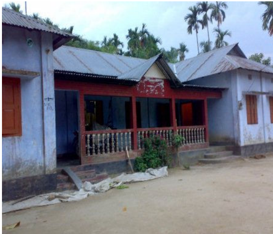
(a) One storey tin shed building.
