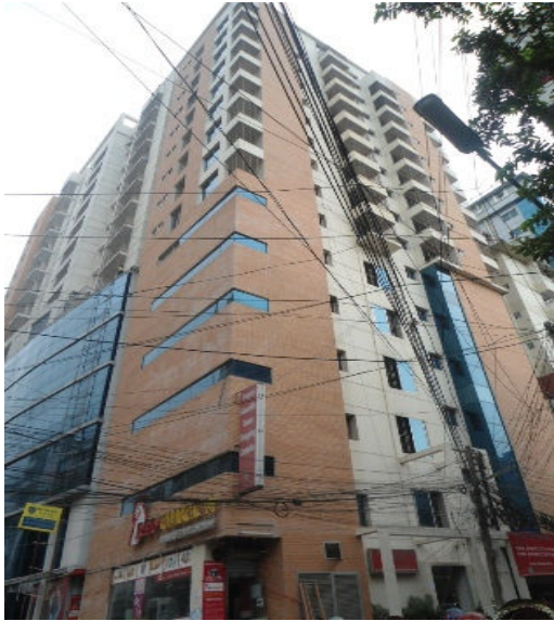
(c) High-rise mostly residential building
