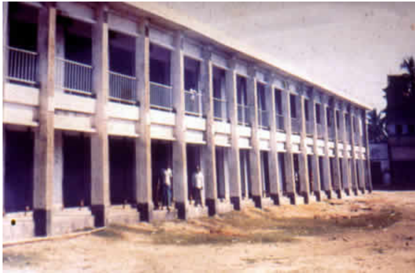
Figure 2.5. Pre-cast Concrete Building.
