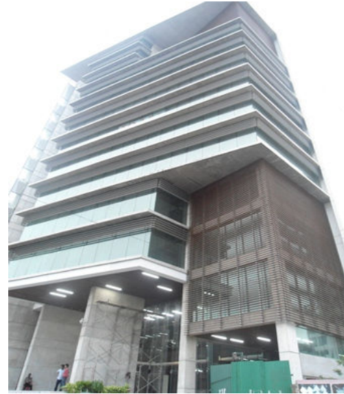
(d) High-rise mostly commercial building
