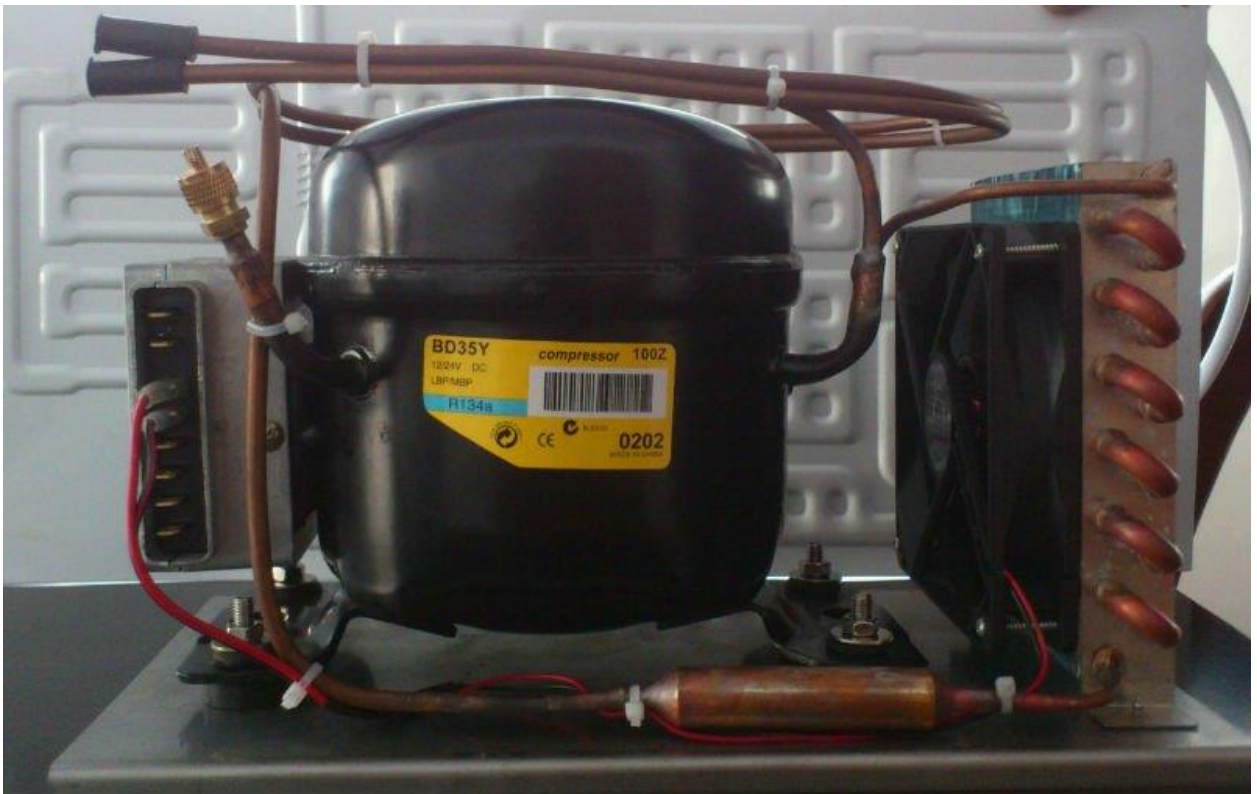
Figure 7: Diagram illustrating the compressor of a system.
