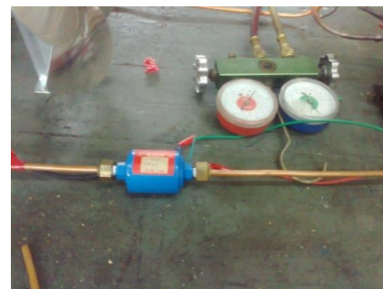
Filter Drier and Pressure Gauge
