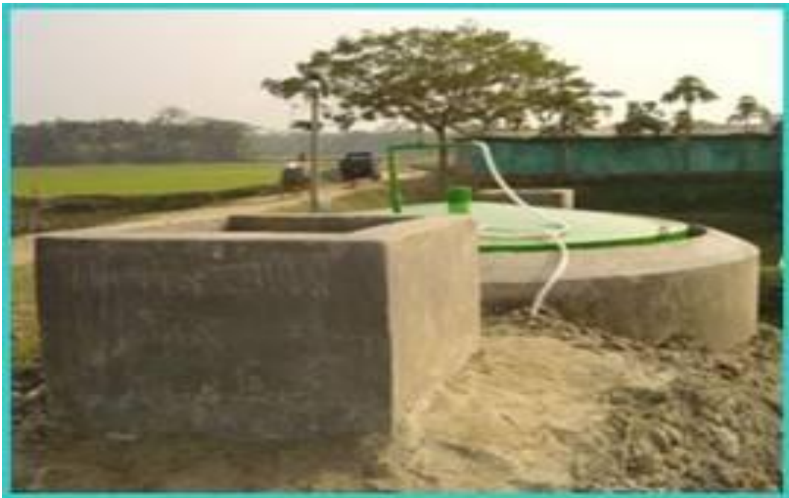
Fig: Biogas Plant
