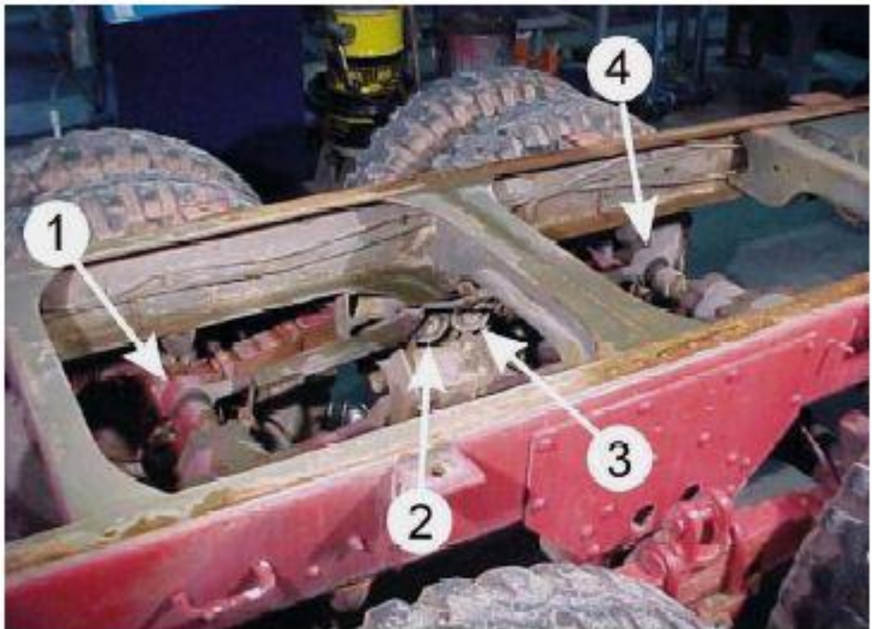
Figure 3. The two upper torque rod assemblies (four rod ends) may be inspected from below the unit. However, for photographic purposes, the water tank was removed from this unit.
