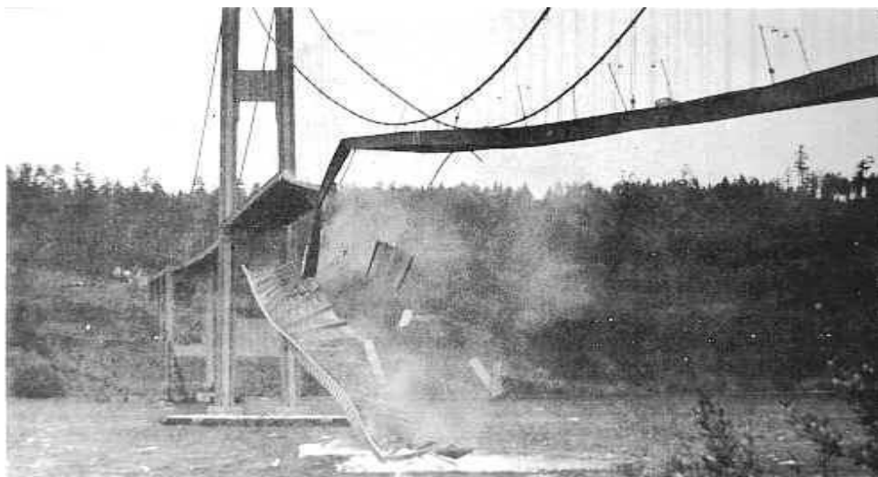
Figure 2.2: Destruction of bridge due to resonance
