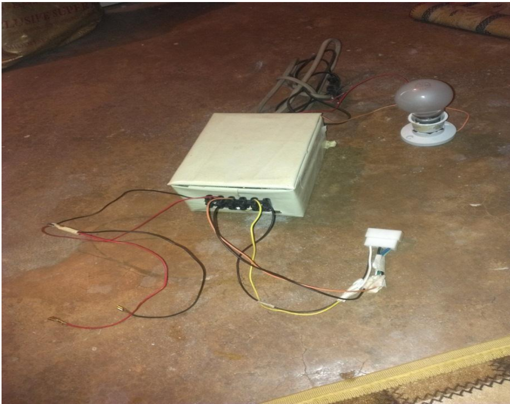
Picture of constructed project with casing
