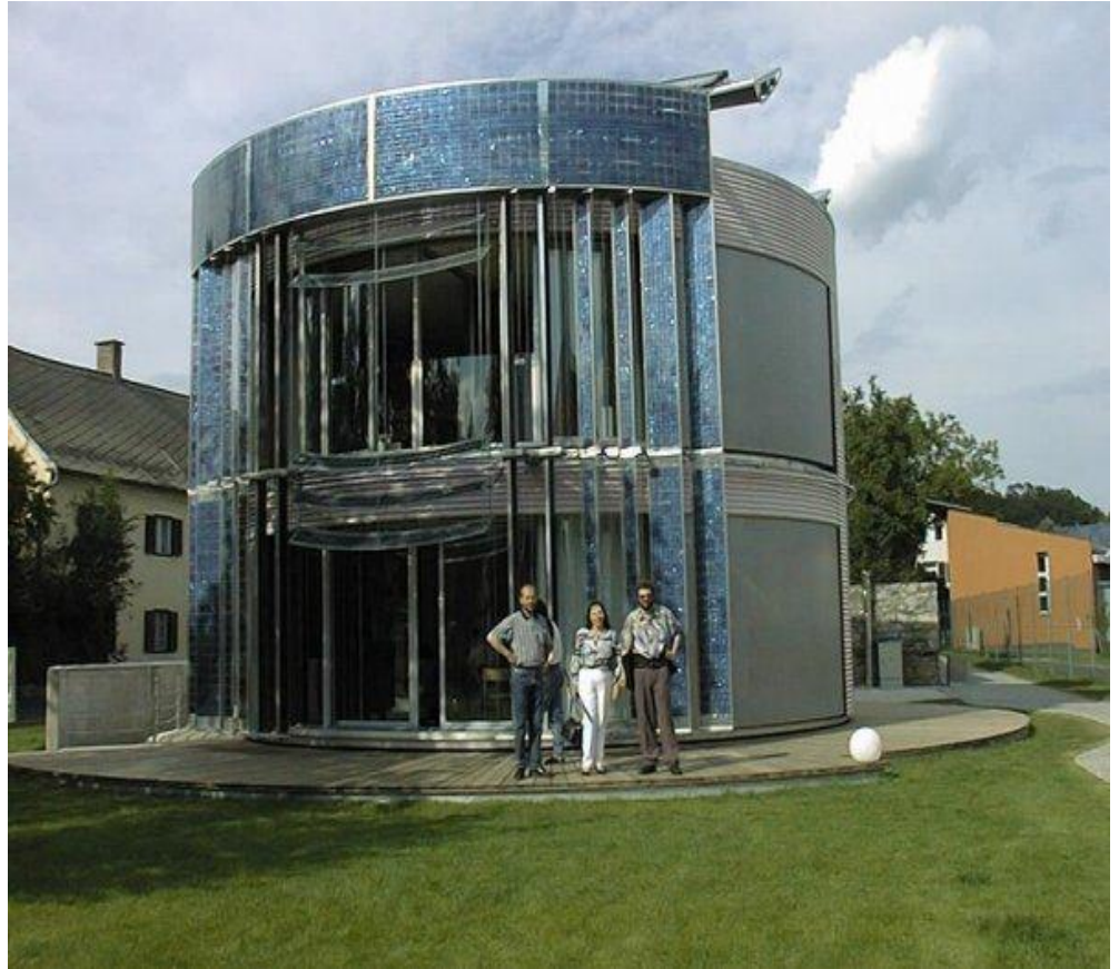
Gemini House rotates in its entirety and the solar panels rotate independently, allowing control of the natural heating from the sun
