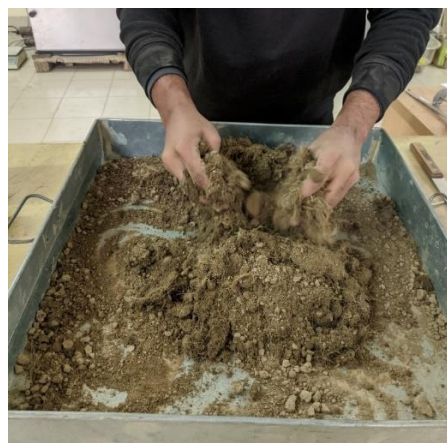
Figure 3.23 Soil, Water & Fiber mixing
