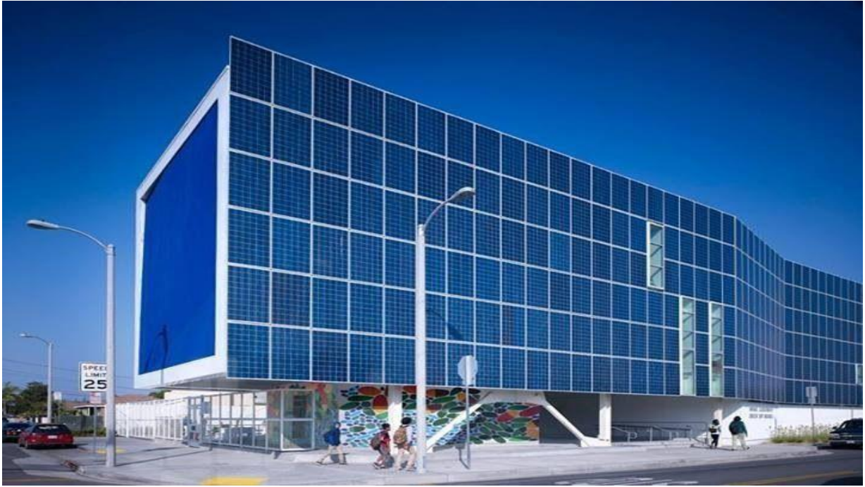
Figure 7: Solar Cell facade building
