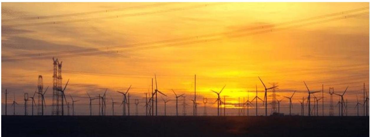
Figure 29: Gansu Wind Farm, China
