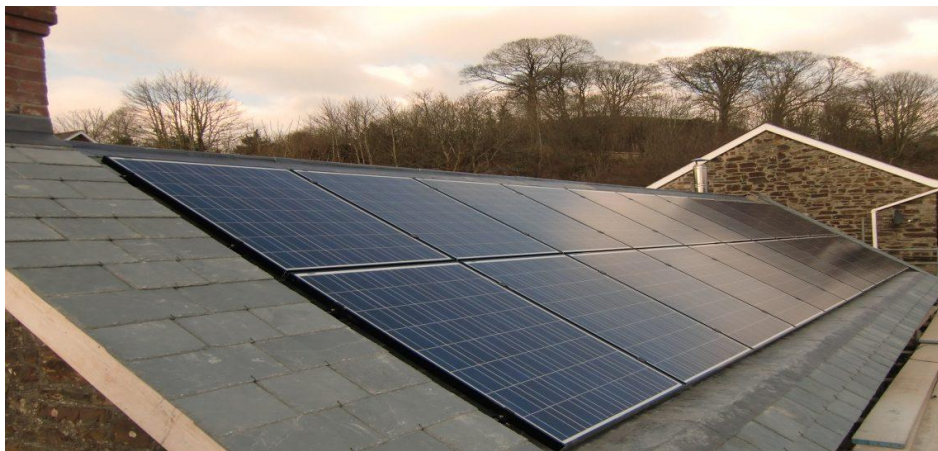
Figure 23: Flush Roof Mounting
