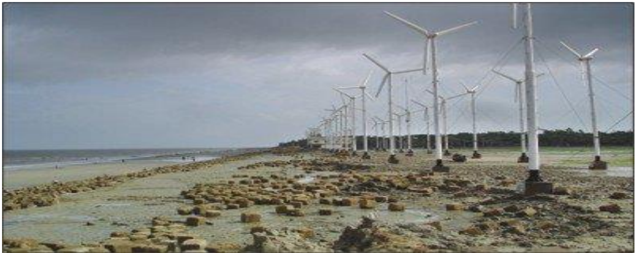
Figure 32: Kutubdia Wind Power Plant
