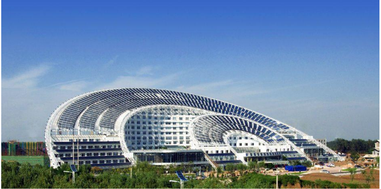
Figure 7: The largest solar power building situated in the northwest of china
