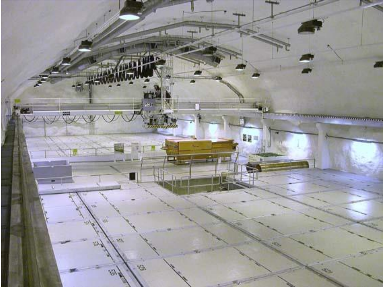
Figure: Low and Intermediate Level Waste Repository at Olkiluoto in Finland (Posiva)
