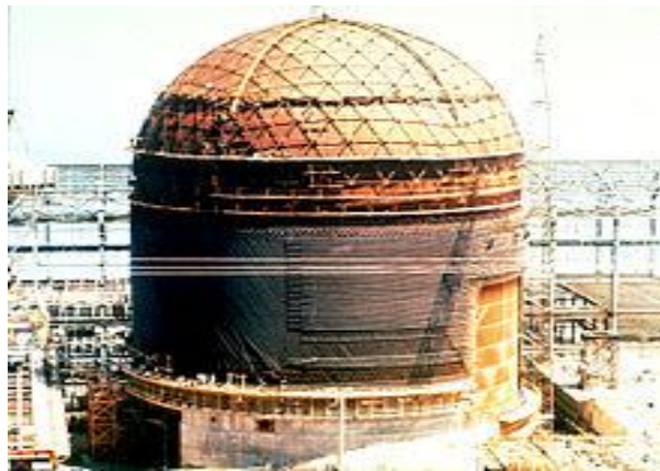
Example of decommissioning work underway
