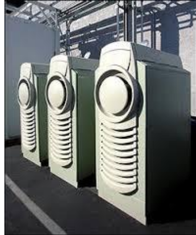
Fig.1.3: Microturbine generators
