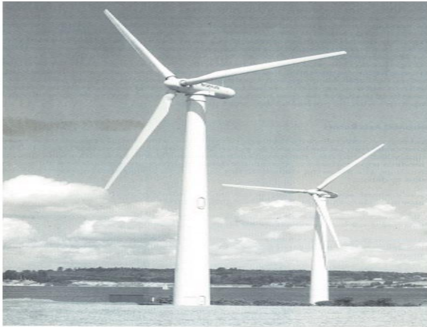
Figure 2.3. A 450 kW HAWT with 37 m rotor diameter [4].
