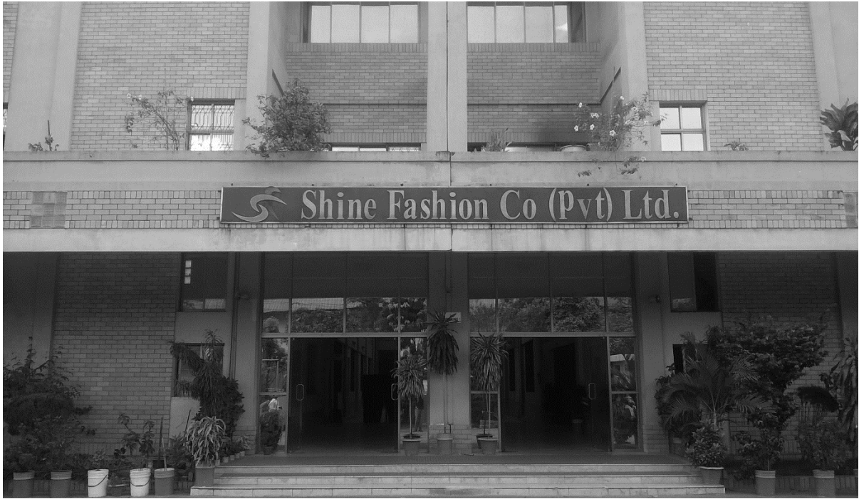
Figure 4.1 : Front Entrance of the Factory
