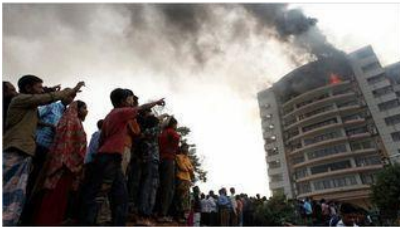
Figure 12: Hamim Group's Factory in blaze, 14 December 2010 (Bilaj, 2010)
