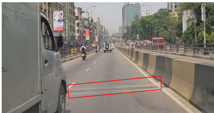
Figure 4-13: Expansion Joints of Mohakhali Flyover
