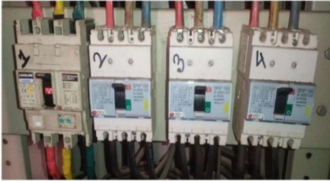
Figure 4.15: Main MCCB (TP) breakers going to 1st,2nd,3rd,4th,5th and dean room of first academic building
