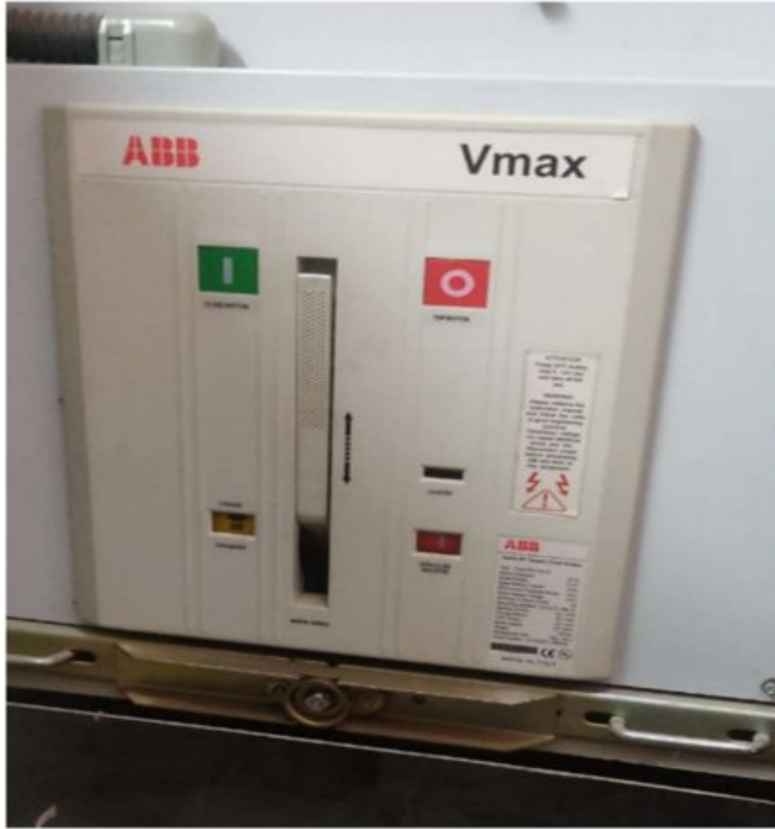
Figure 4.4: Vacuum Circuit Breaker used at the HT side with nameplate
