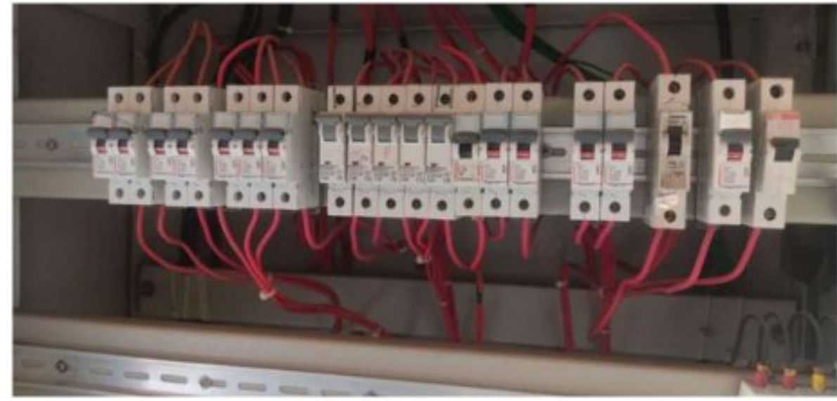
Figure 4.16: Other MCCB (TP) and MCB (SP) circuit breakers coming from the LT panel to the first academic building
