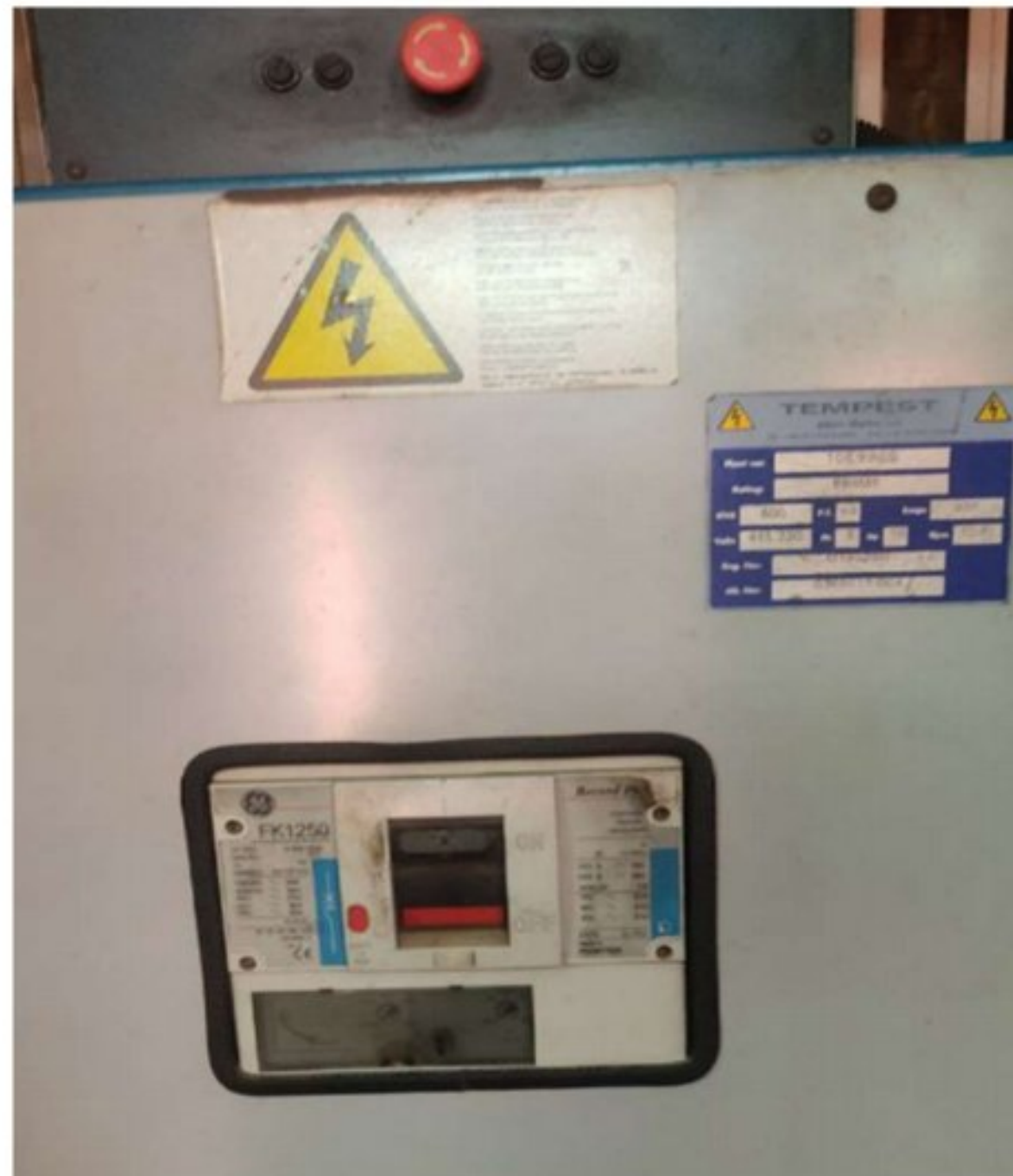
Figure 4.7: The 615 kVA generator of Perkins
