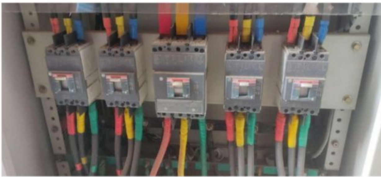
Figure 4.16: Other MCCB (TP) and MCB (SP) circuit breakers coming from the LT panel to the first academic building
