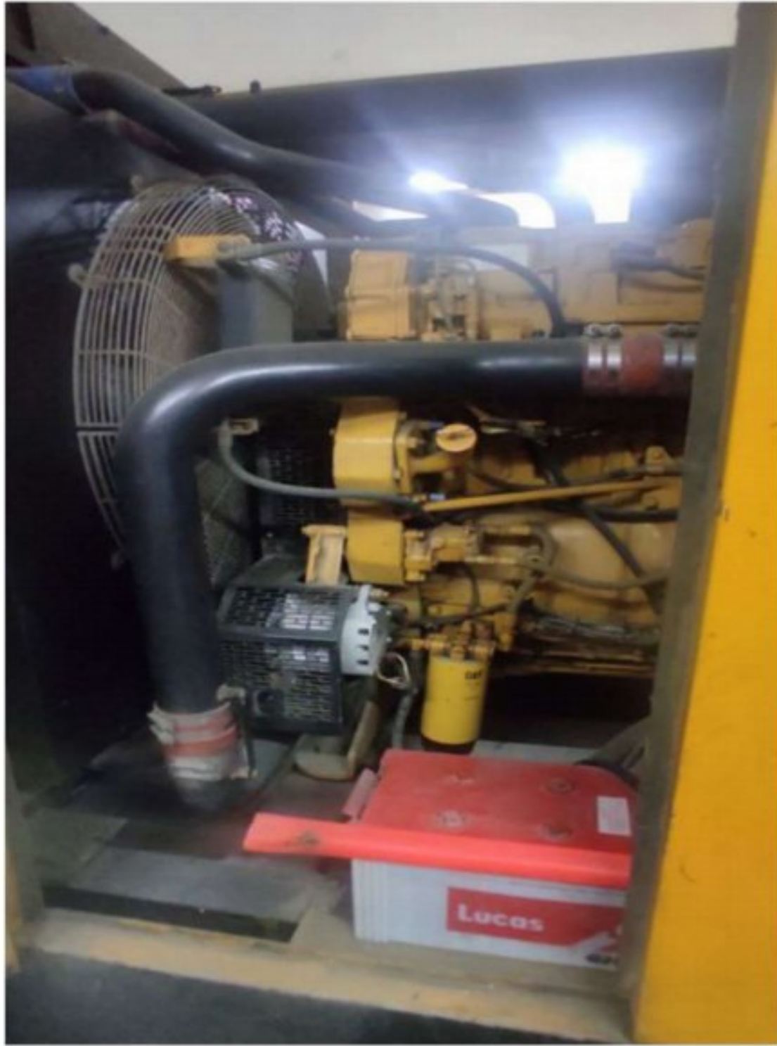
Figure 4.6: The 635 kVA generator of caterpillar along with the nameplate
