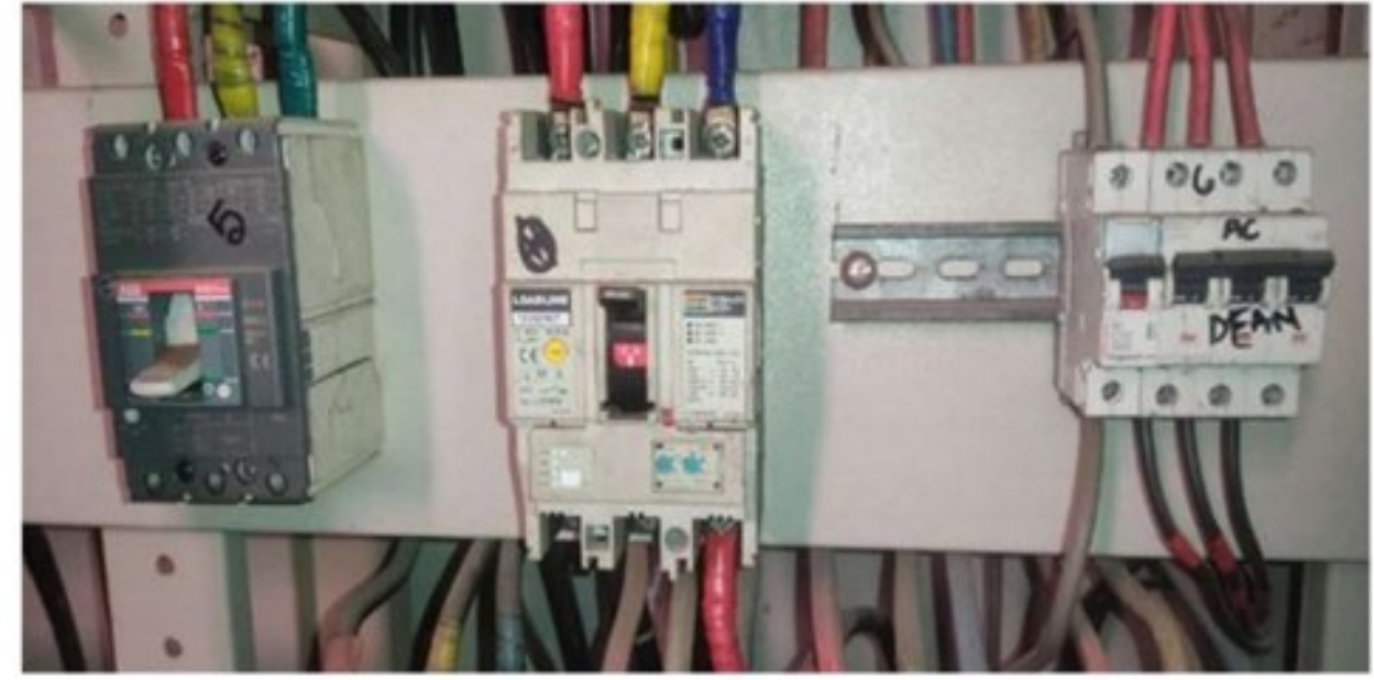
Figure 4.15: Main MCCB (TP) breakers going to 1st,2nd,3rd,4th,5th and dean room of first academic building
