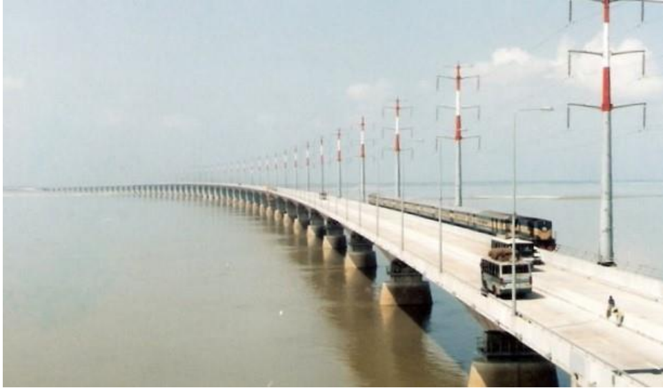
Figure 1.3: Bangabandhu Jamuna Bridge Bangladesh
