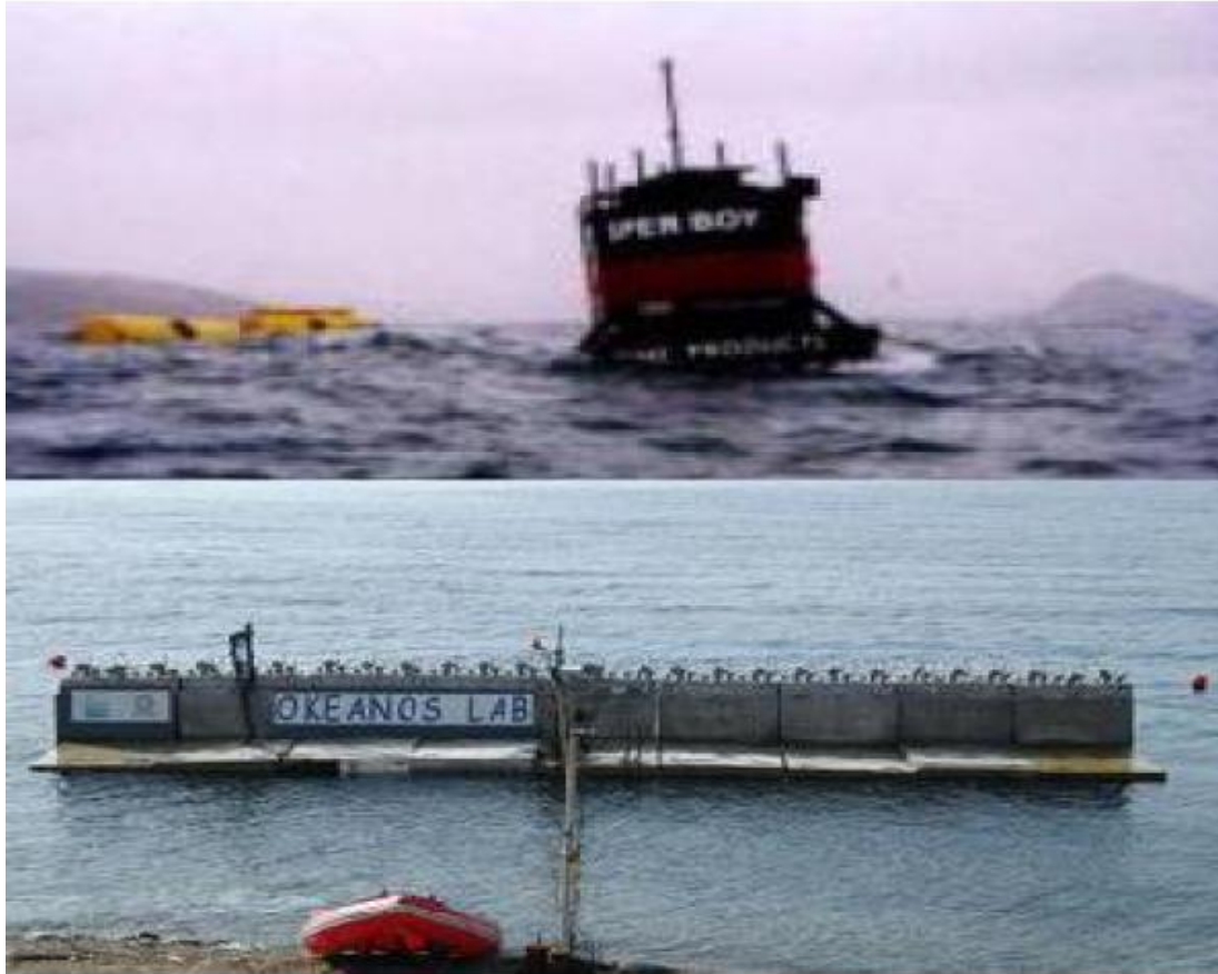
Figure 4: Different concepts of oscillating water columns - Sperboy (above) and REWEC-3 (below) [10]
