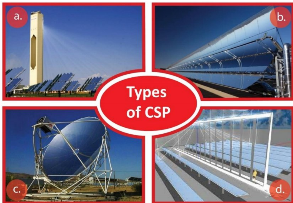
Figure 5: The most common types of CSP technology; (a) SPT, (b) PTC, (c) PDC, (d) LFR
