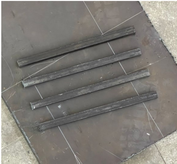
(a) Columns cut to size
