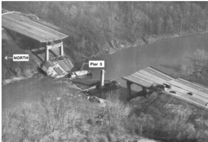
Figure 2.3: Schoharie Creek Bridge Collapse [16]
