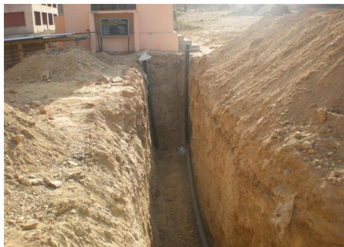
Figure 8: Experimental setup of EATHE system[42].
