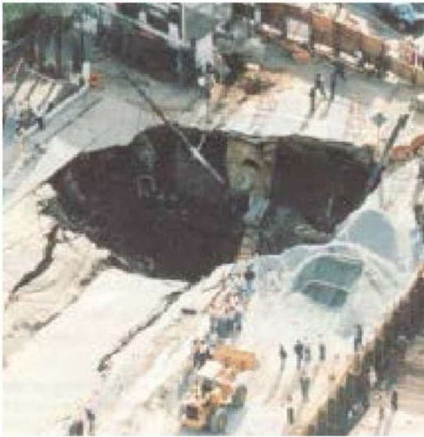
Figure 1.1 Tunnel collapse in Sao Paulo (Neto et al., 2002)
