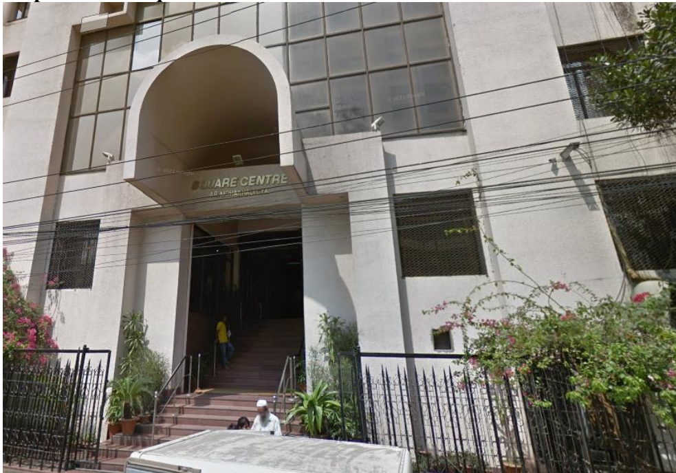
Figure 1 Outside view of corporate headquarters situated at Square Center, 48 Mohakhali C/A
