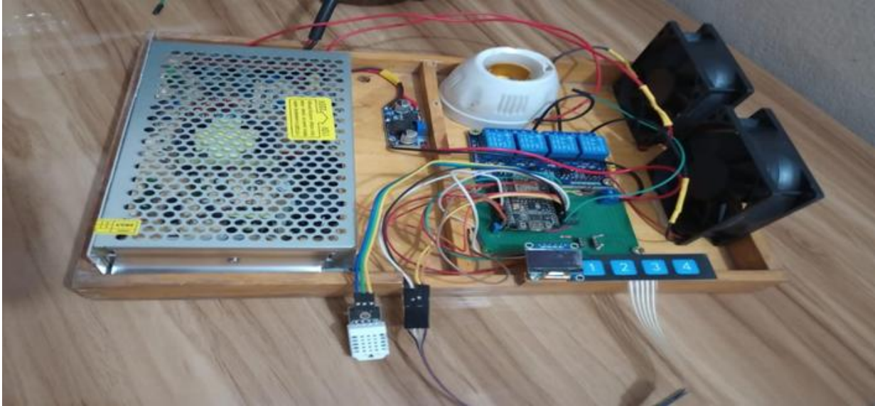
Figure 3.6: Electrical set up for the constructed solar dryer
