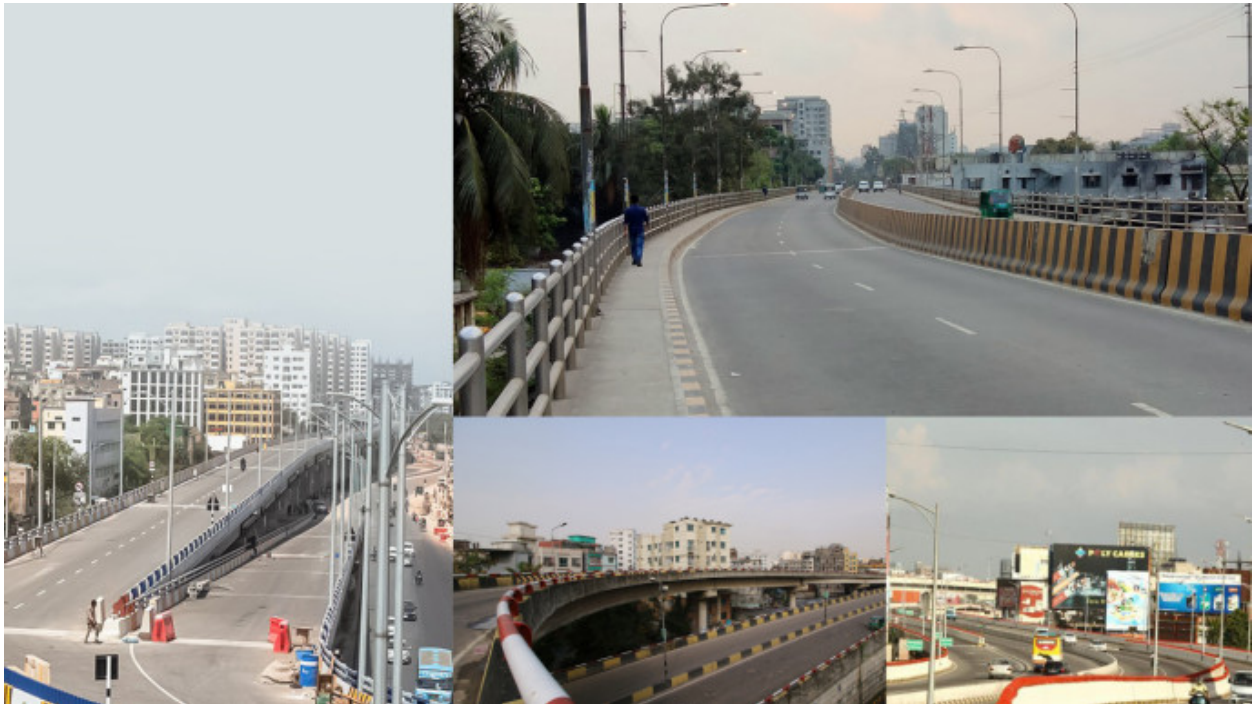
Figure 4.2: Flyovers in Dhaka City
