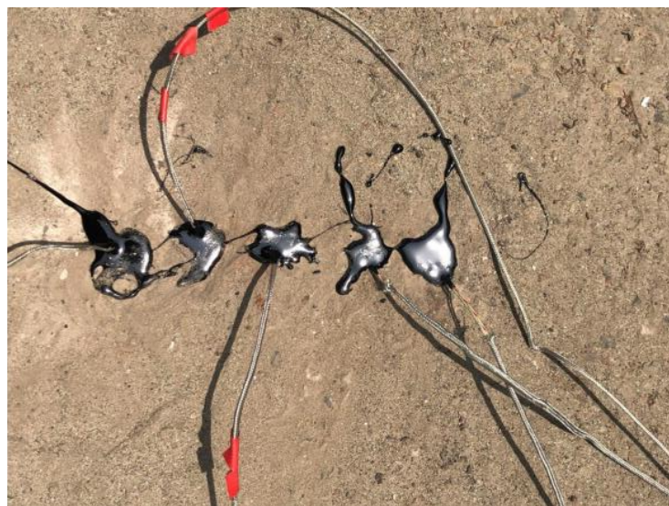
Figure 18: Sealing the holes with bitumen
