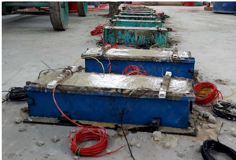
Figure 9: Casting of concrete specimens
