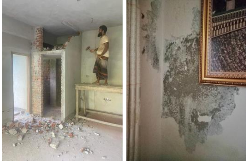
Figure 1: Construction Site (Plastic Paint)
