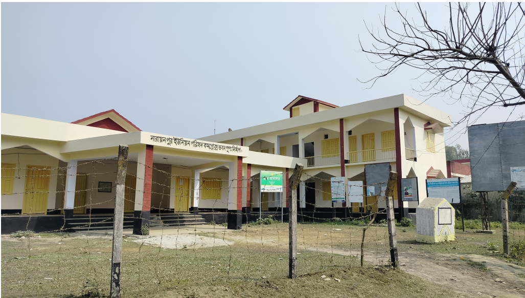
Figure 11: The Inactive Health Centers (Source:Field Visit)
