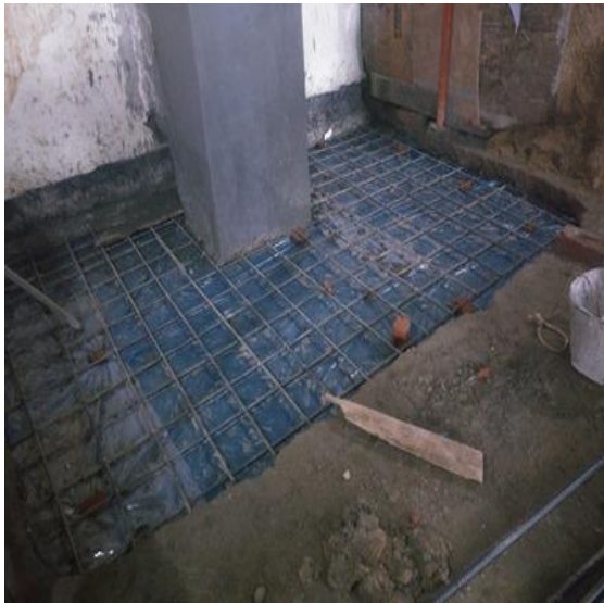
Fig. 5.7: Foundation Retrofitting
