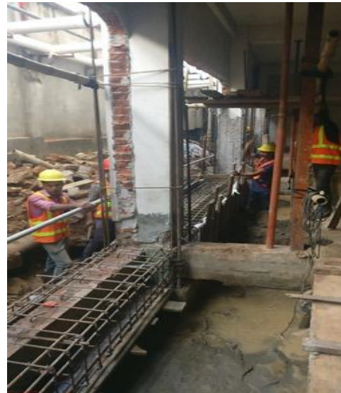
Fig. 5.8: Grade Beam Retrofitting
