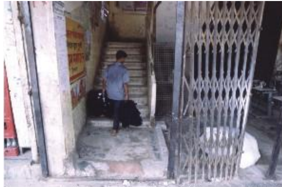
The gate was locked by volunteers' of a religious group that held a programme in the adjacent ally.
