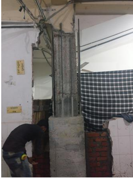
Fig. 5.6: Column Retrofitting
