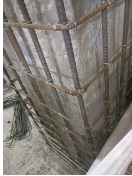
Fig. 5.6: Column Retrofitting
