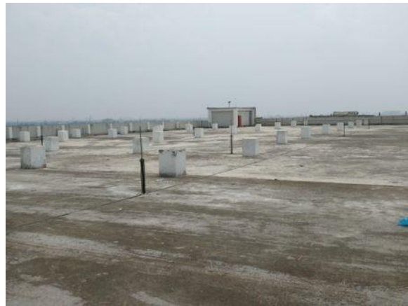
Fig. 5.19: Lightning Protection System (LPS)
