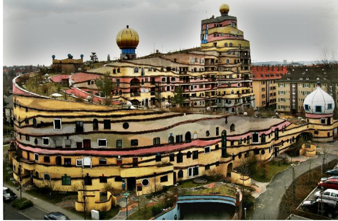
Figure 2.23: Complex of residential buildings “Waldspirale”, Darmstadt, Germany
