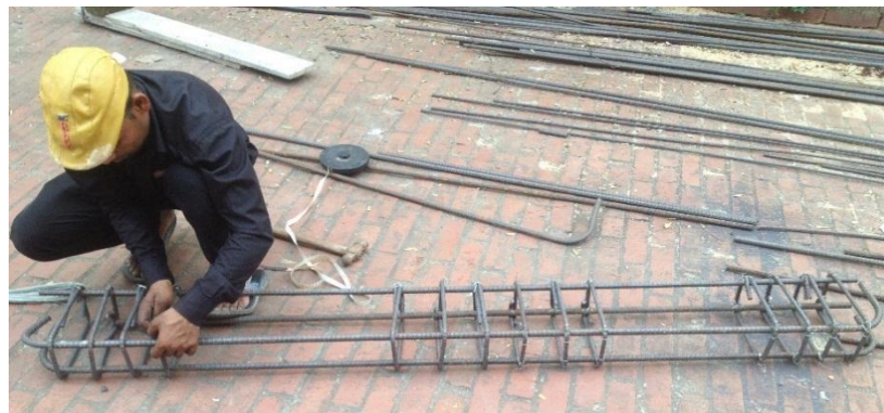
Figure 3.10: Preparing Reinforcement case
