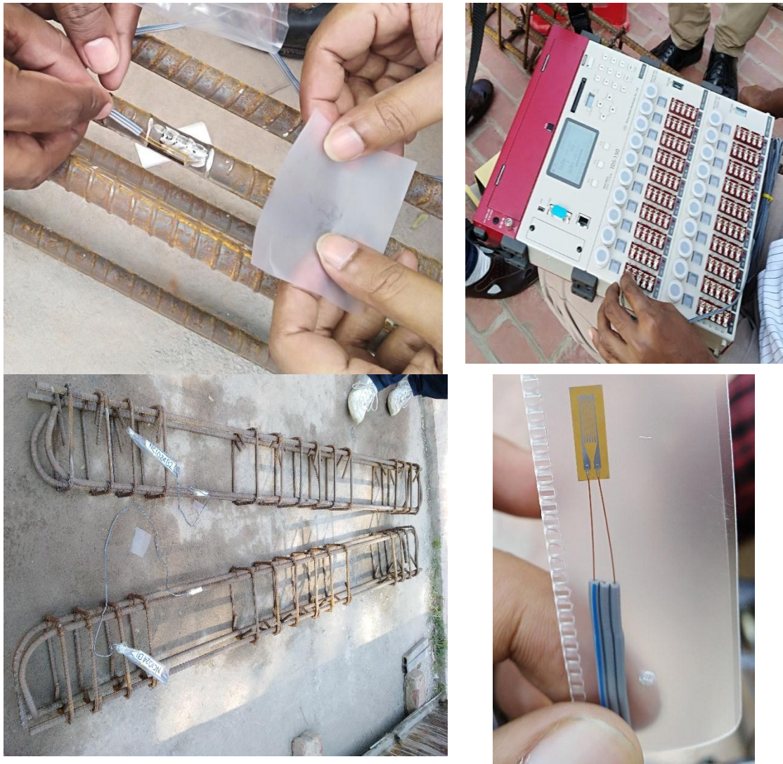
Figure 3.14: Installation of the strain gauge and datalogger
