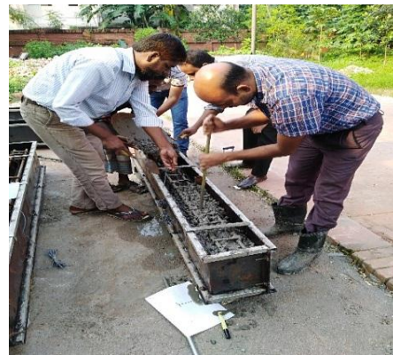
(b) Concrete Placement
