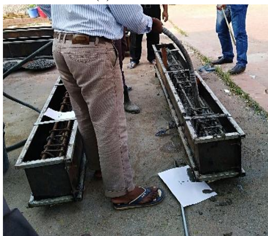
(c) Concrete consolidation
