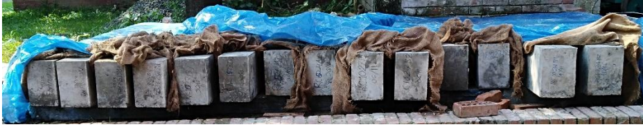
Figure 3.12: Curing of casted beams
