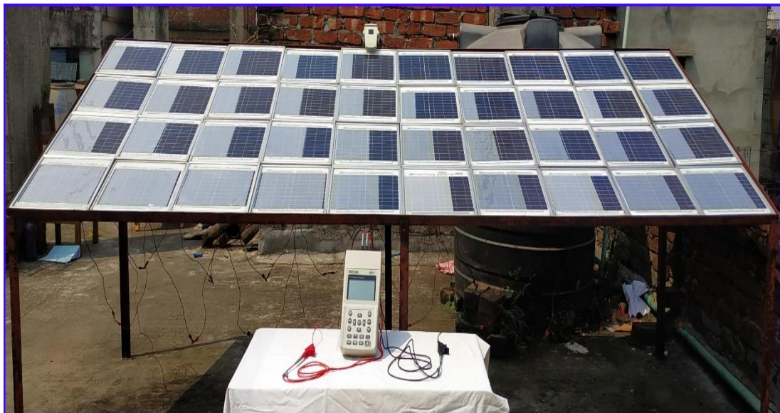
Figure 3.9: Experimental setup of the non-uniformly aged PV array (front view)
