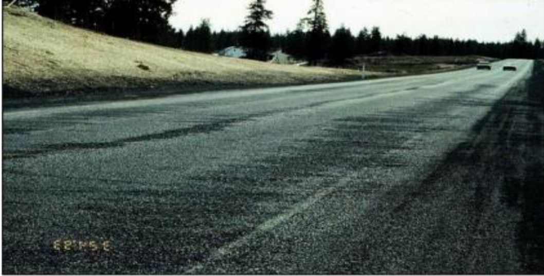
Figure: Effect of stripping distress on HMA pavement layer.
