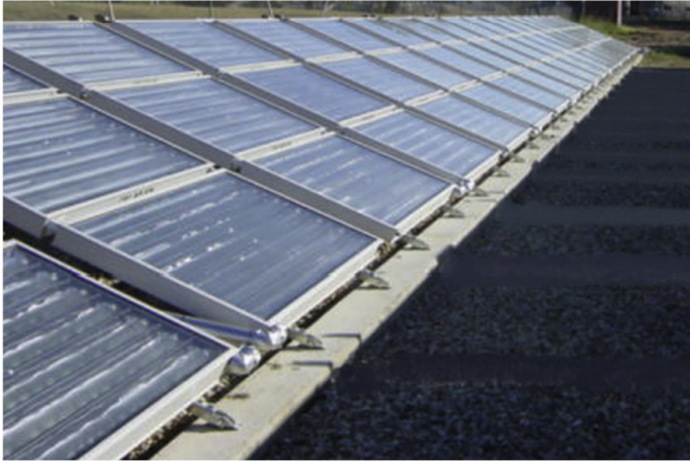
Figure 3.8: Photo of a CPC panel collector installation of panel CPC collector with cylindrical absorbers [30]
