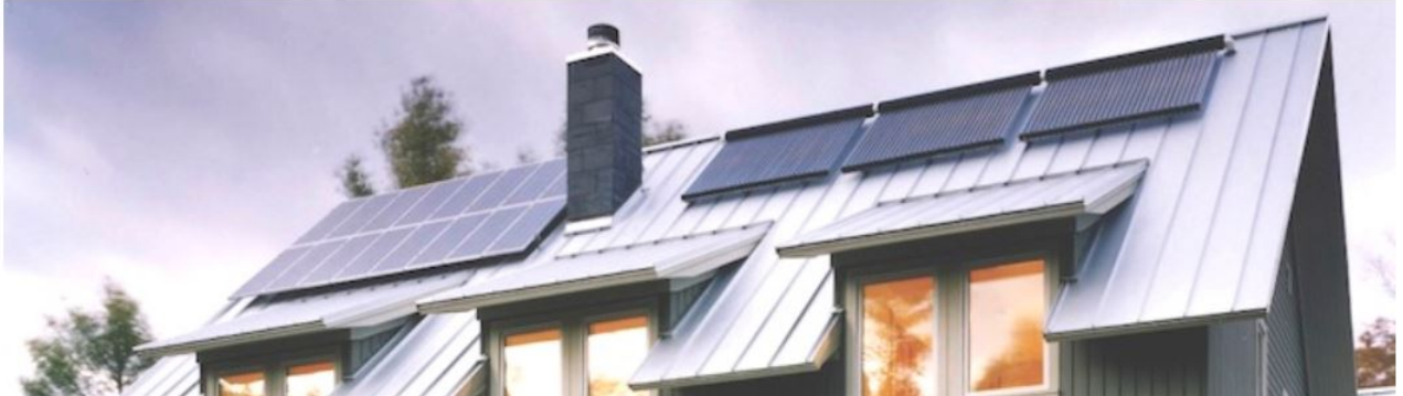
Figure 3.3: A system that incorporates a solar thermal system with a modest sized PV system is a great option.
