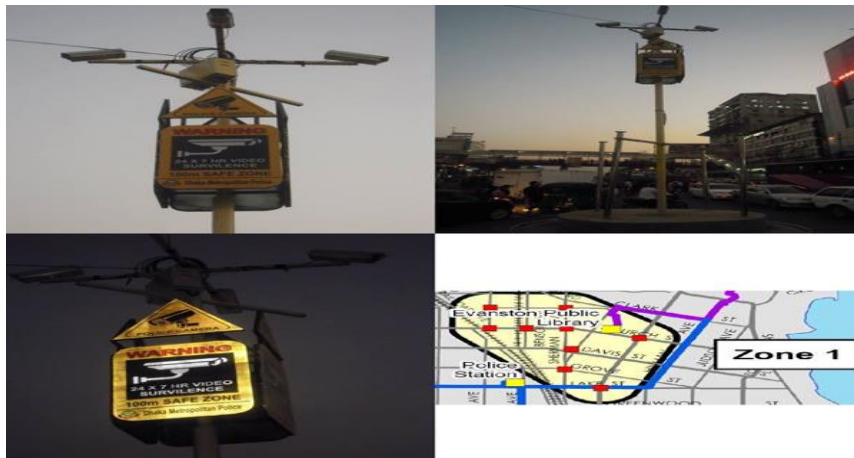
Figure 4-32: Surveillance Camera Presence
