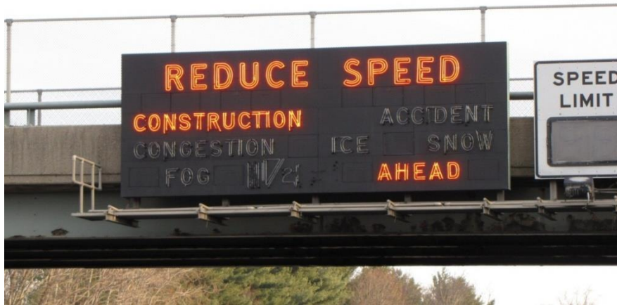
Figure 4-33: Variable Message Sign
