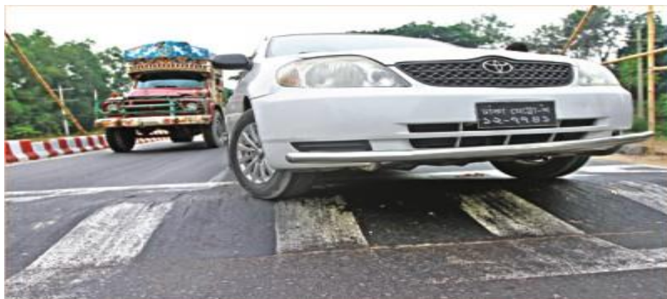
Figure 4-8: Presence of Speed Breaker
