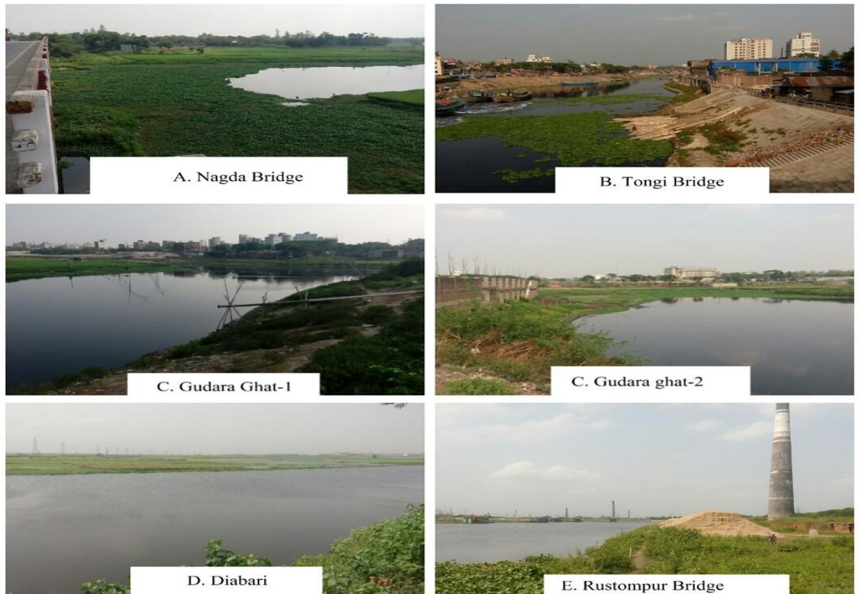
Figure 2.2: Pictures of the Site
