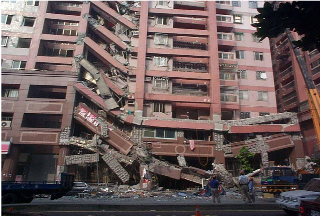
Fig 1.1: Structural Damage in 1999 Taiwan earthquake.
