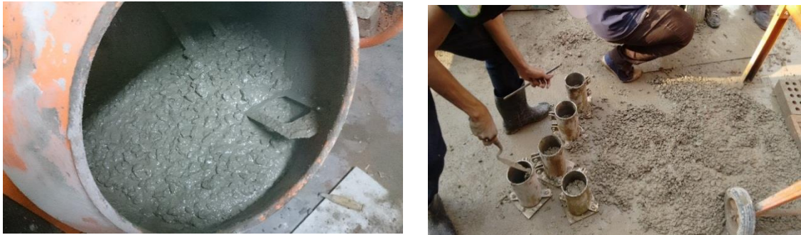
Photo 3.9 Mixing & Casting of Concrete
