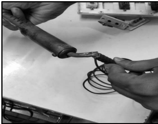
Connecting Electric Cables
